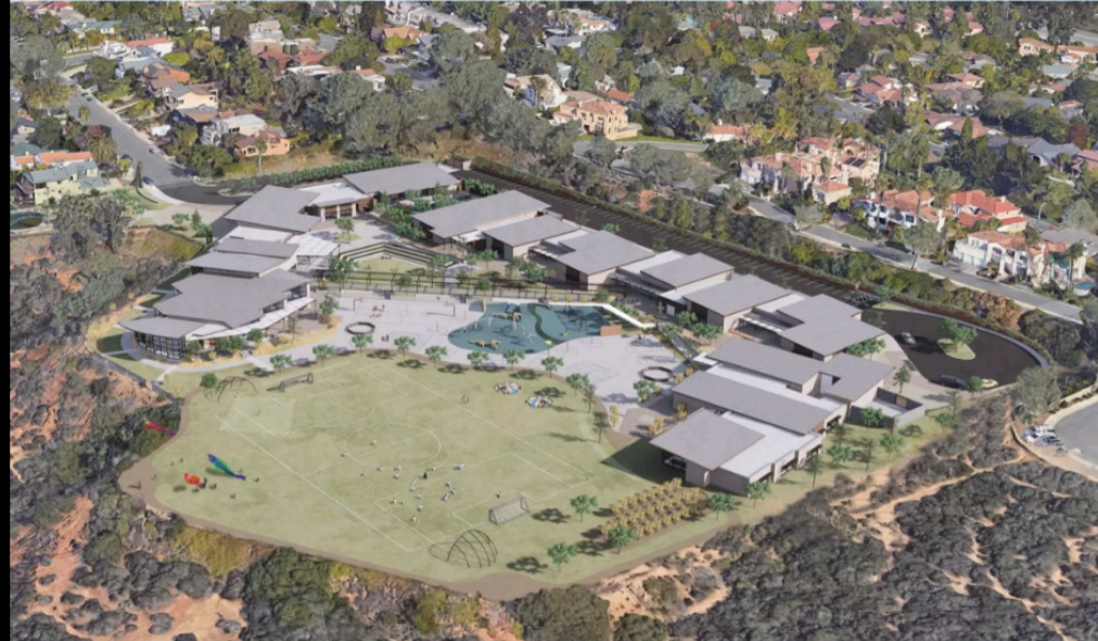
DEL MAR HEIGHTS SCHOOL REBUILD
